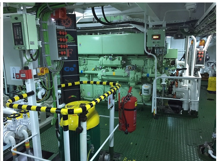
Engine Room Lower Floor
